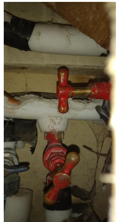
Fig. 2 and 2a: Domestic Stop Cocks Blue = mains water supply; Red = drain valves
