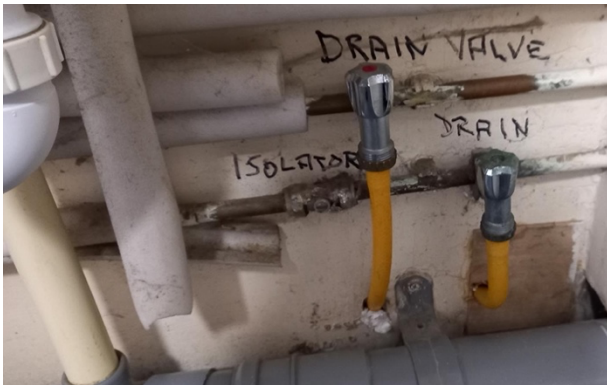
Fig. 3: Toilet Drain Valves
