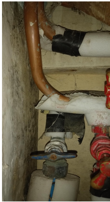
Fig. 2 and 2a: Domestic Stop Cocks Blue = mains water supply; Red = drain valves
